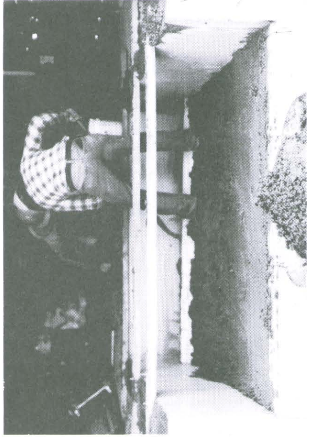
REMODELING - HANG THE PERMA PIT FROM THE FLOOR, BRACE IT AND SINGLE POUR.
