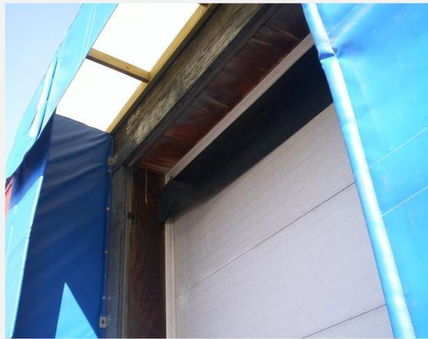
*Rigid head frame is peaked to prevent snow and water build-up and covered with white vinyl to allow light in.*
